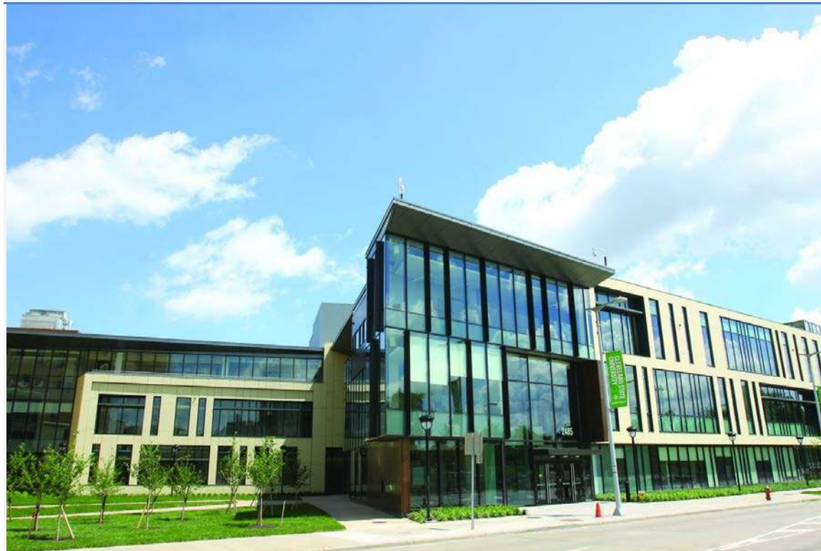
Figure 5.1 Outfitting a New Building
